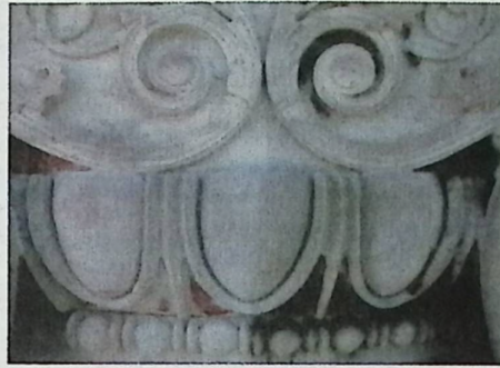
Fig. 14. Cleaning for the removal of black crust.
